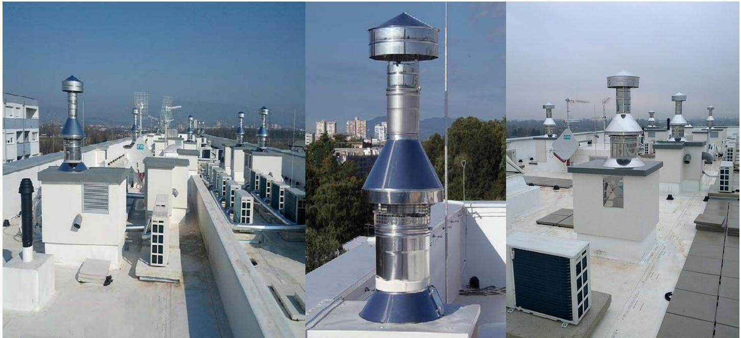
***BONOS® CLS KOAKSIJALNI SISTEM DIMNJAVA ZA PLINSKO GRIJANJE
